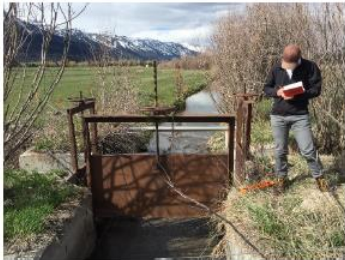
Photo 24 Three-way Headgate, Prosperity Ditch at Highway 22
