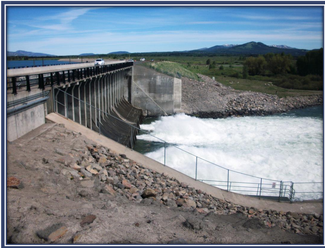
JACKSON LAKE DAM OUTLET WORKS
