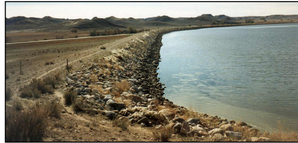
Healy Reservoir dam
