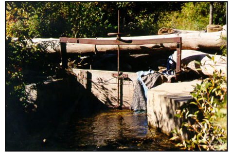
Garrard Ditch headgate
