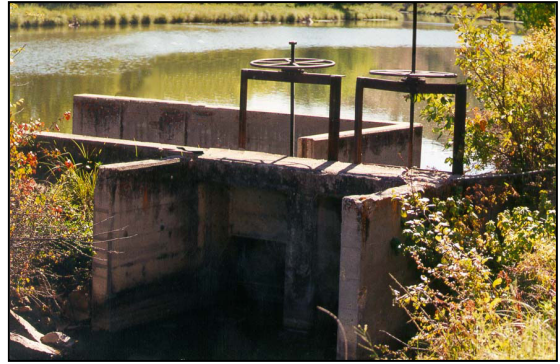
Interstate Ditch headgate
