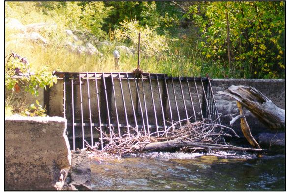
High Line Ditch headgate
