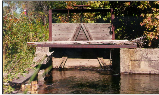
South Side Ditch headgate
