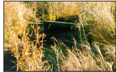
Mowry Basin flume
