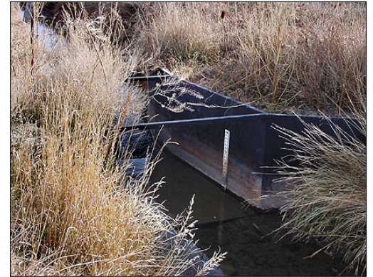
Prince Albert Ditch flume
