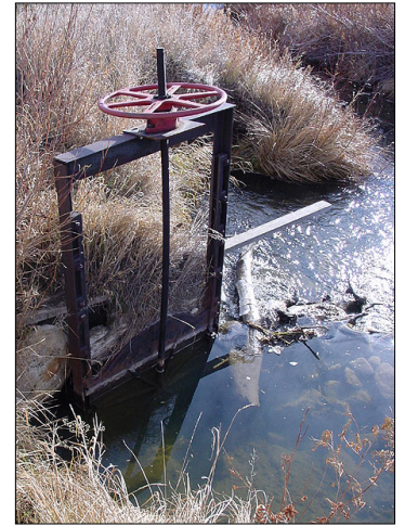
Prince Albert Ditch headgate
