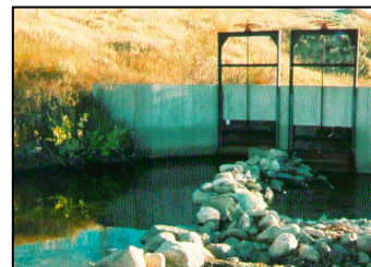
Lake DeSmet Ditch headgate
