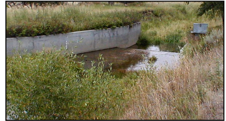
Leiter Ditch Flume
