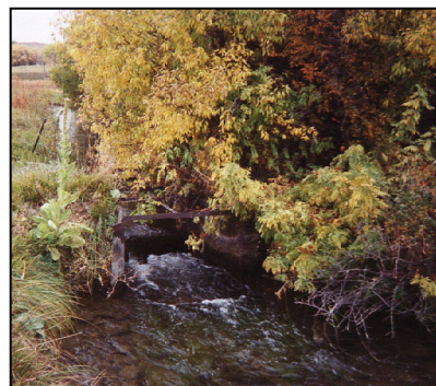
Dunlap Ditch Flume
