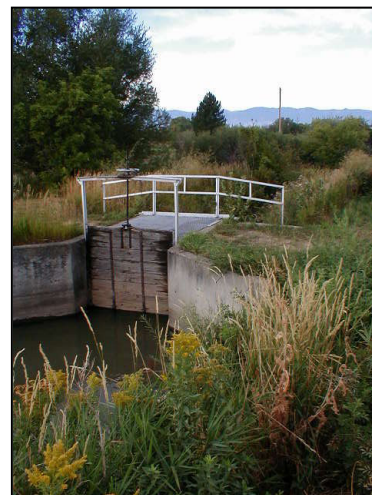
Burn Cleuch Ditch Headgate
