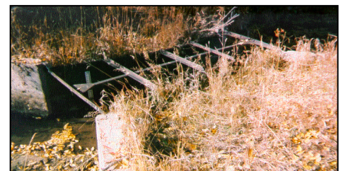
Penrose Ditch at Johnson Creek flume
