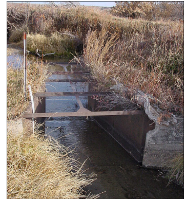
Hopkins Ditch flume
