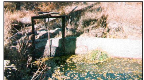
Penrose Ditch at Johnson Creek headgate
