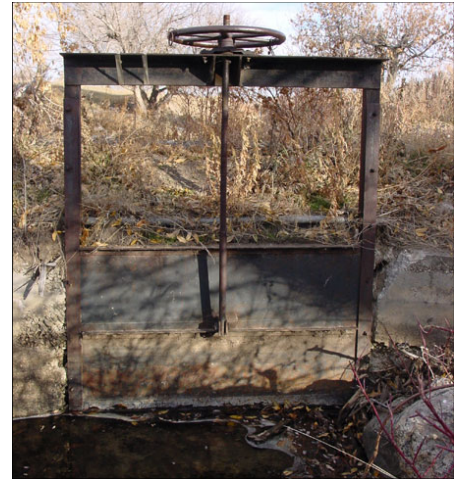
Hopkins Ditch headgate
