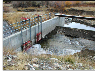
Cook Ditch Headgate
