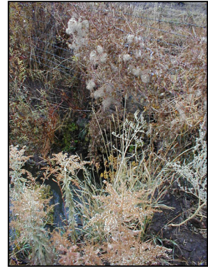
Thompson Brothers headgate
