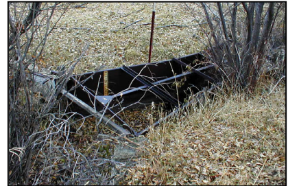
North Fork Diversion Flume
