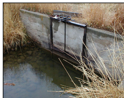
PX Ditch Headgate
