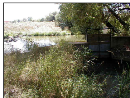
Grinnell Ditch Headgate & Dam
