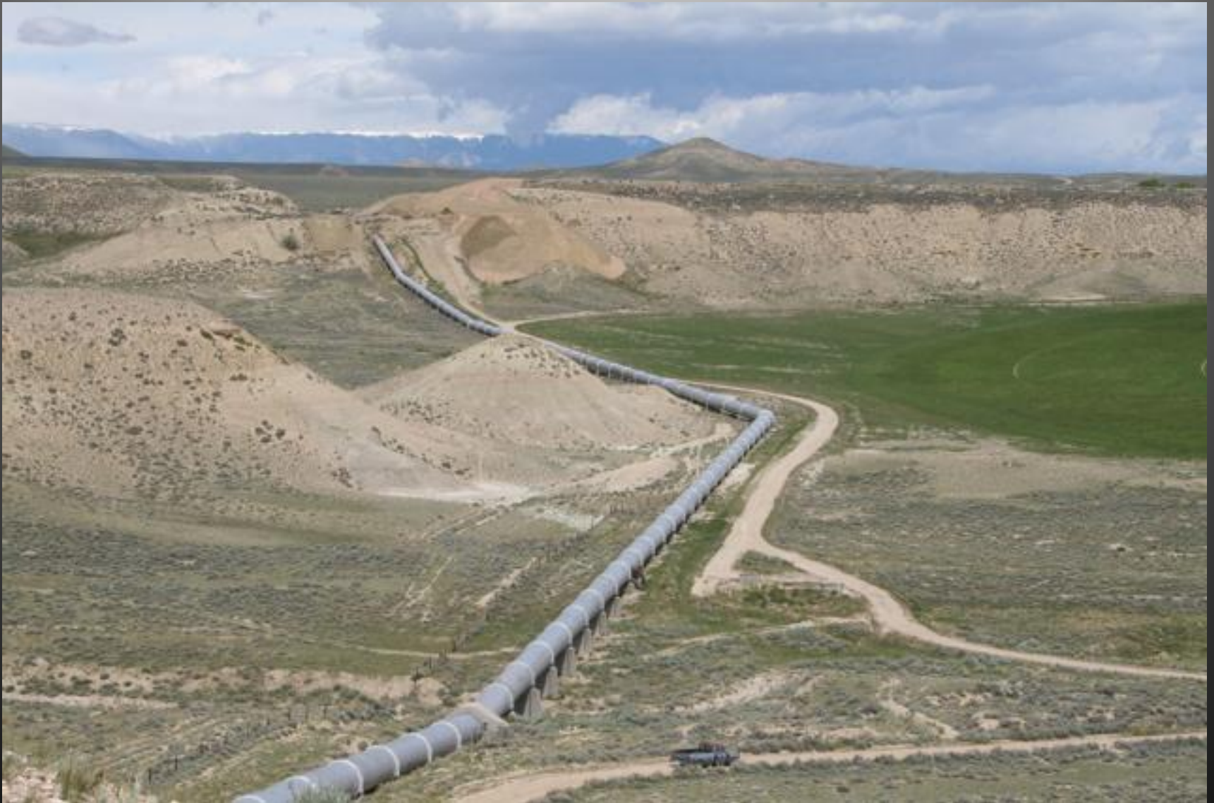
Heart Mountain Irrigation District
