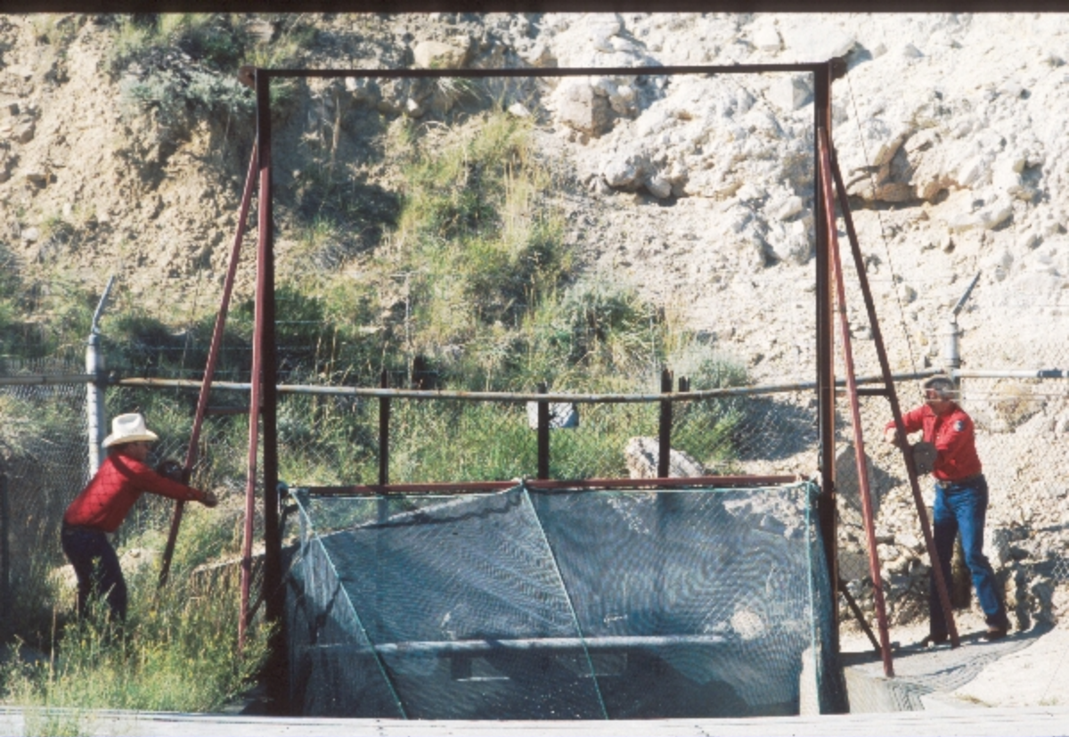
Sieve Net at terminus of Shoshone Conduit—Heart Mountain canal
