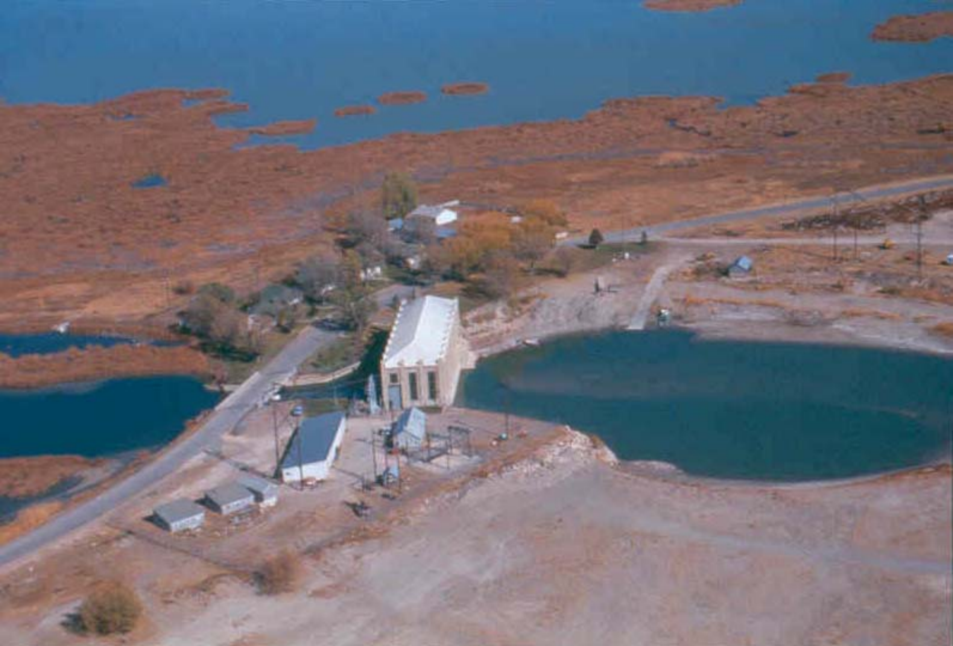
LIFTON PUMPING PLANT
