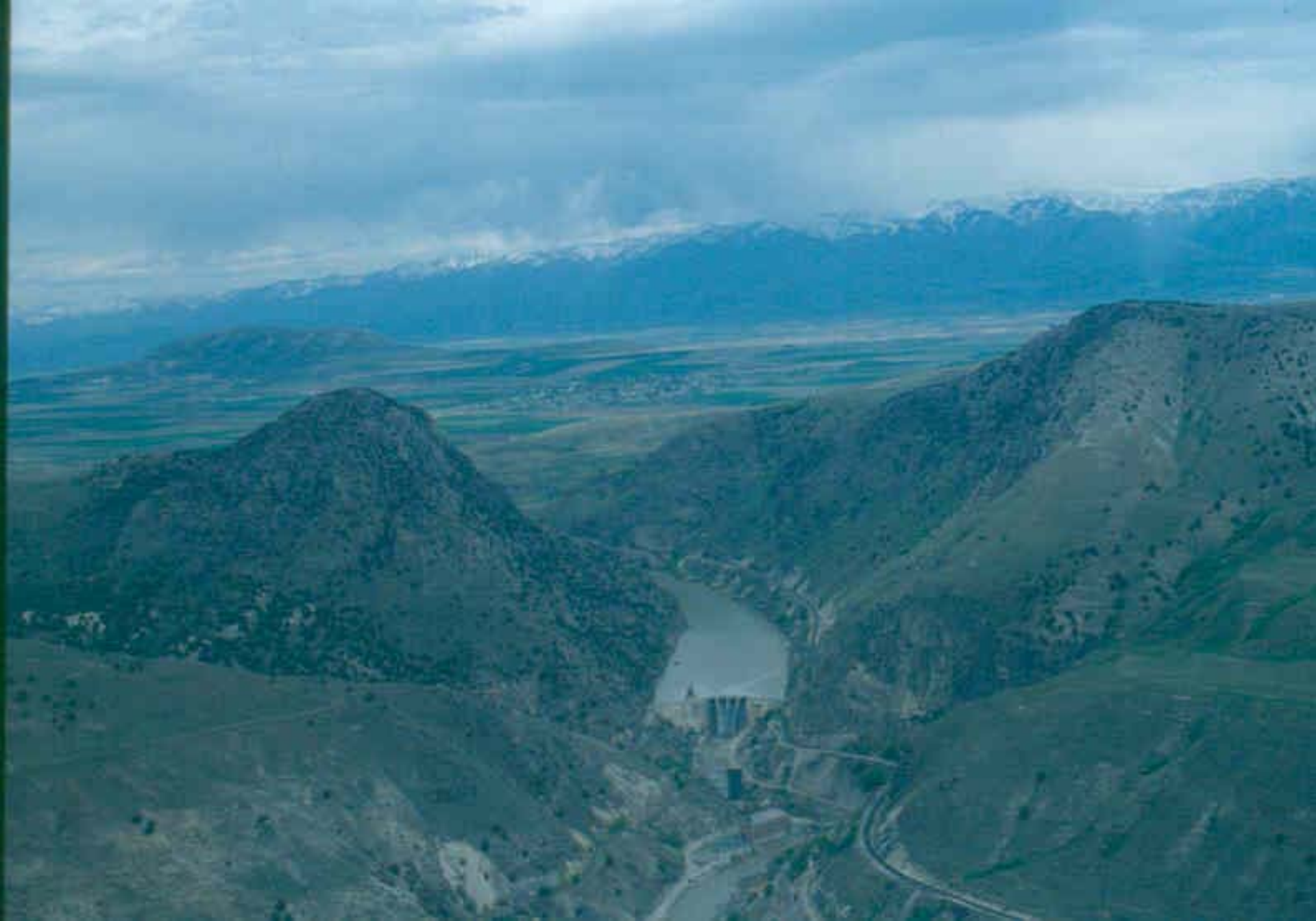
CUTLER DAM & RESERVOIR
