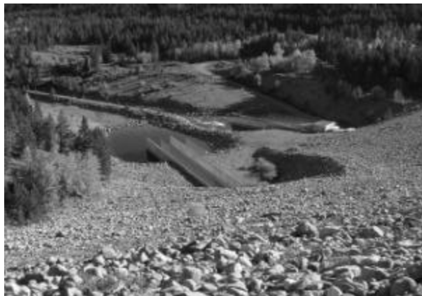
Meeks Cabin Dam
