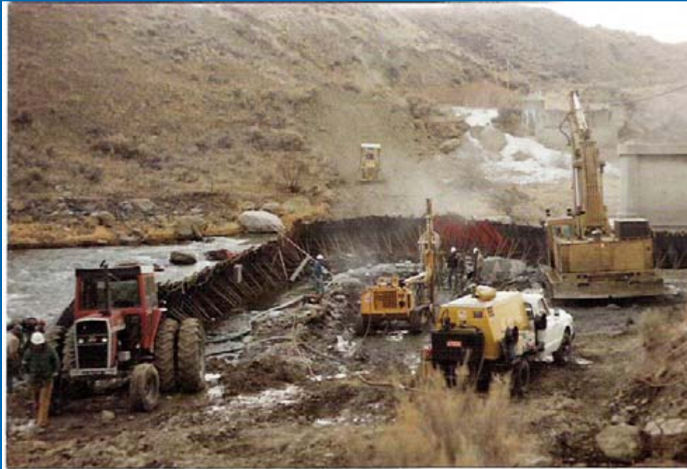
PORT-A-DAM HOLDING BACK THE SHOSHONE RIVER
