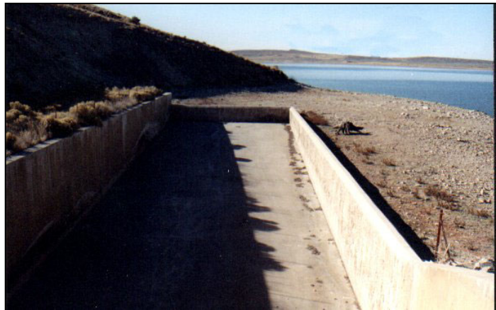
Woodruff Narrows Spillway
