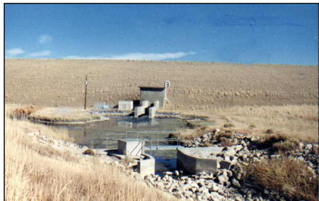
Sulphur Creek Outlet Structure
