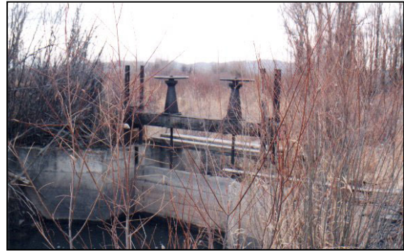
Whites Water headgate structure
