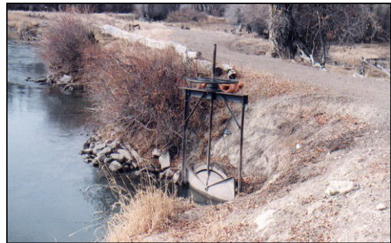
South Branch Irrigating headgate structure
