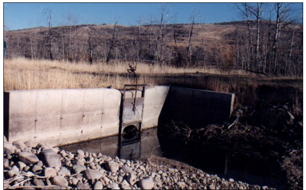
Myers Irrigation diversion headwall
