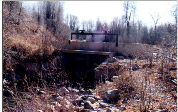
Hilliard West Side diversion structure
