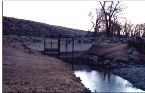
Francis Lee headgate
