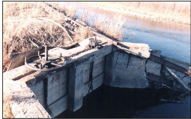
Evanston Ditch Headgate
