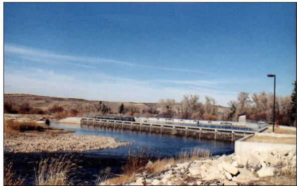
Evanston Intake Facility on the Bear River
