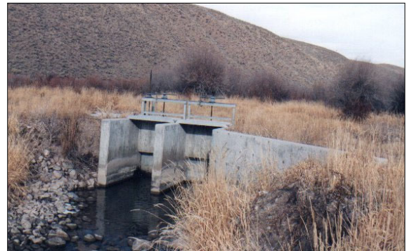
Covey Canal headgate structure
