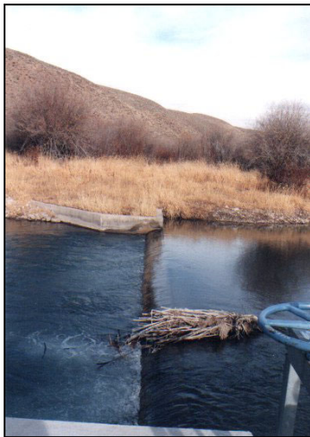
Covey Canal cut-off wall across the Smiths Fork
