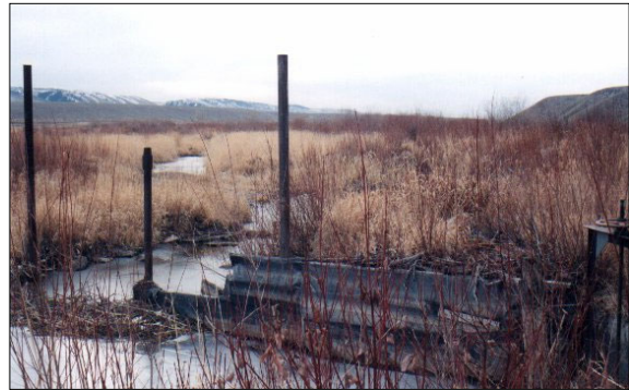
Cooper Ditch headgate structure
