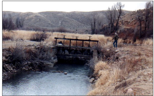
Cook Brothers headgate structure
