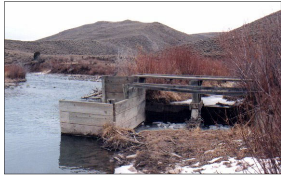
Button Flat headgate structure
