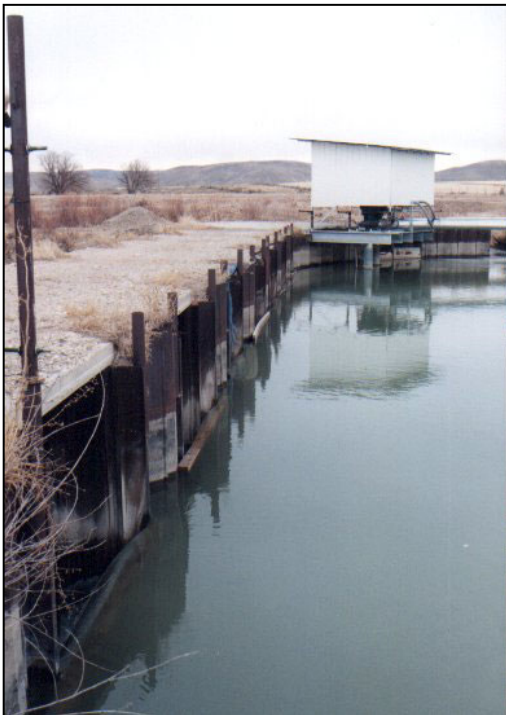
Upstream side of B.Q. dam (looking east) - Weston Ranch Pump facility can be seen at the back near the east bank
