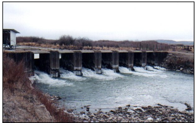
Downstream side of B.Q. Dam structure
