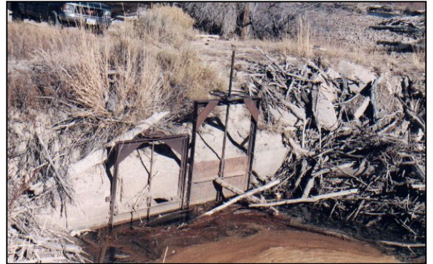
Booth Ditch headgate
