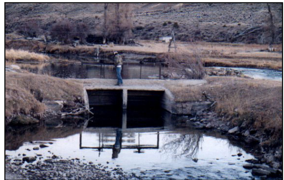
Bear River Canal headgate
