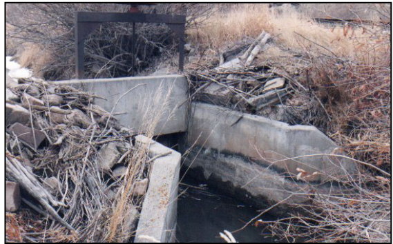
Alonzo F. Sights headgate structure
