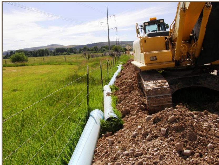
Installation of the Evanston Bear River Regional Pipeline, 2009
