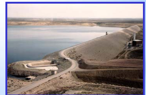
Fontenelle Dam and Reservoir
