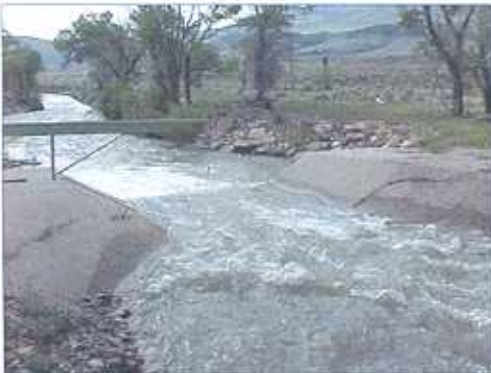
Gauging Station, above Anchor Dam on South Fork Owl Creek
